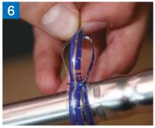
Remove pressing indicator. Check the correct insertion depth has been met.
